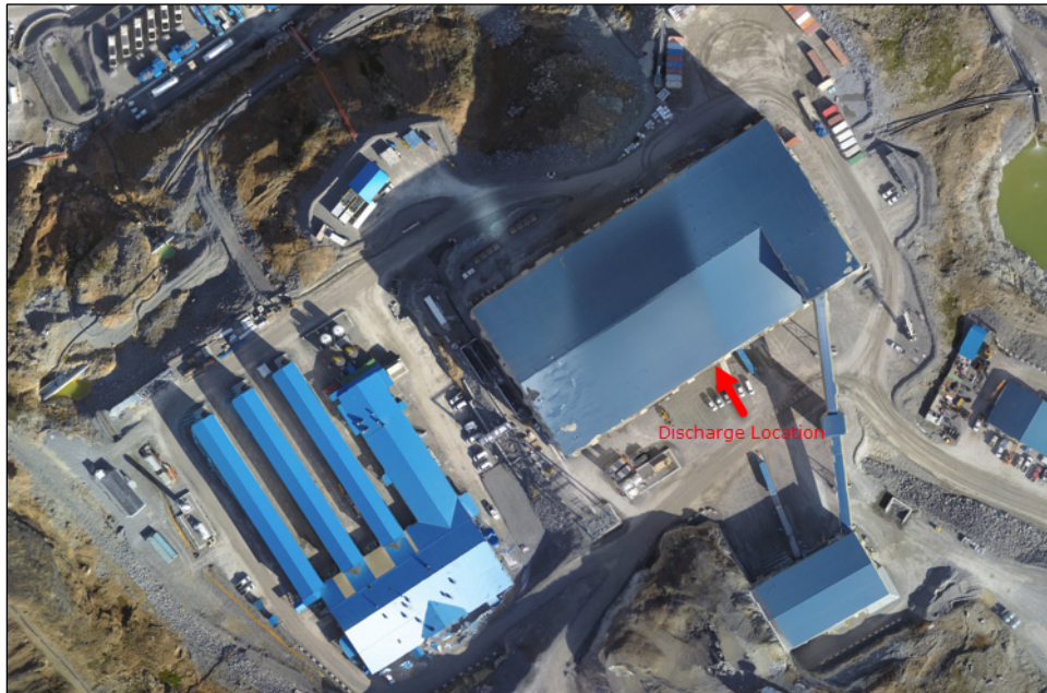
Figure 2.2-6: The Proposed Discharge Location for the Core Saw Exhaust, on the Southeast Side of the Mill
